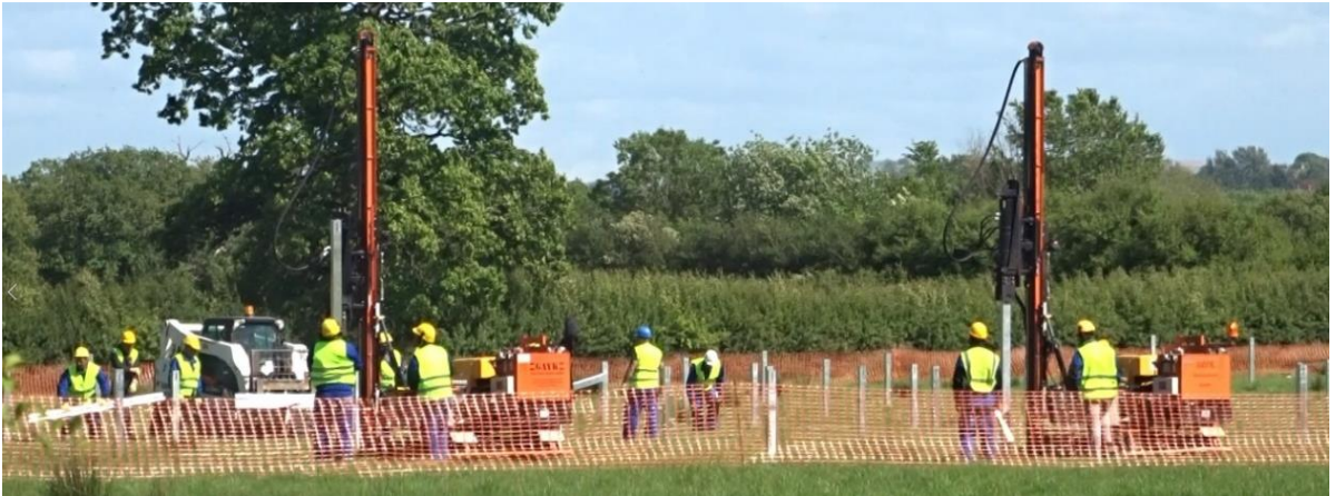
Photograph 14.9: Framework Posts being Installed (Bentham Farm, July 2015)
