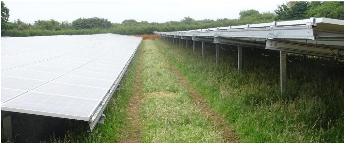
Photograph 14.11: After Solar PV Panels Bolted-on (Bentham Farm, August 2015)
