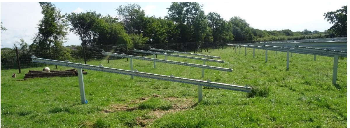
Photograph 14.10: Framework Posts Installed (taken at Bentham Farm, July 2015)
