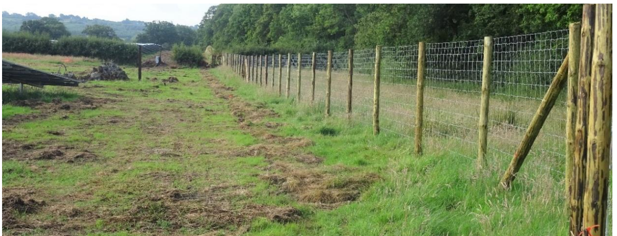
Photograph 14.15: The Location of Photo 14.15 Two Weeks Later
