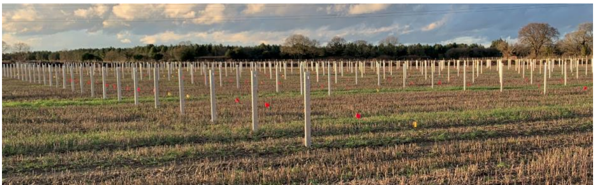
Photograph 14.8: Recently Installed Framework Posts (Tiln Farm, Retford, January 2023)
