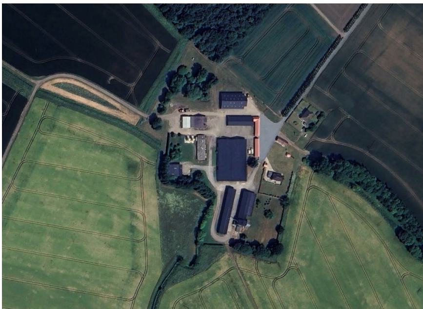
Plate 9 2023 Google Earth image of Quosquo Hall showing removal of more of the building – the last remnant of the southern range is gone.
