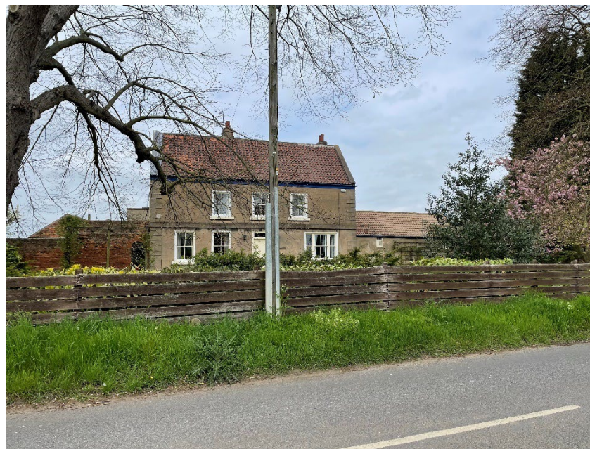
Plate 19 View of Manor Farmhouse from the road looking north
