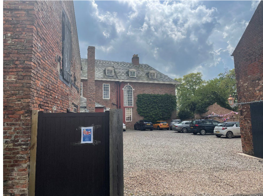
Plate 14 View of rear (north facing) façade of Camblesforth Hall and service yard
