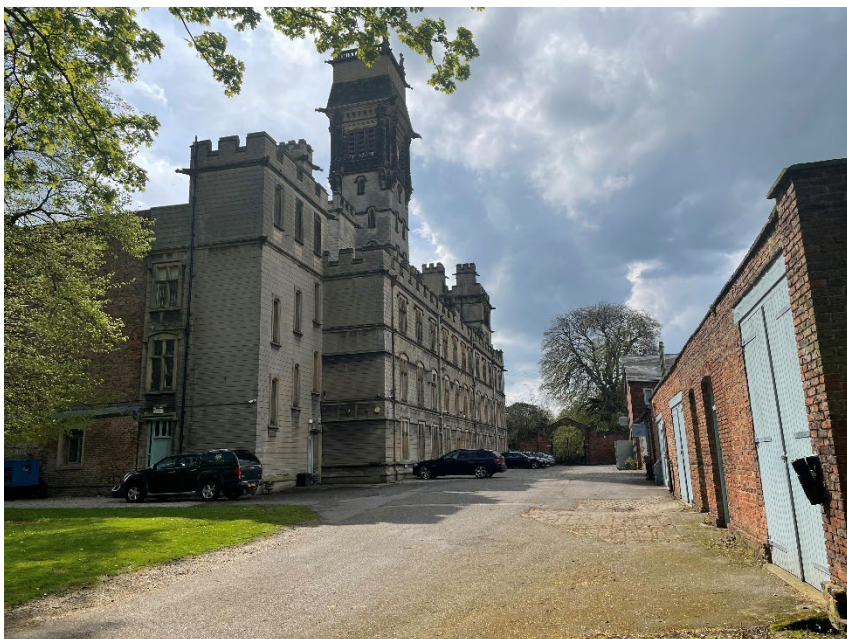
Plate 17 View looking west of the main body of Carlton Towers with stable-block and vineyard opposite
