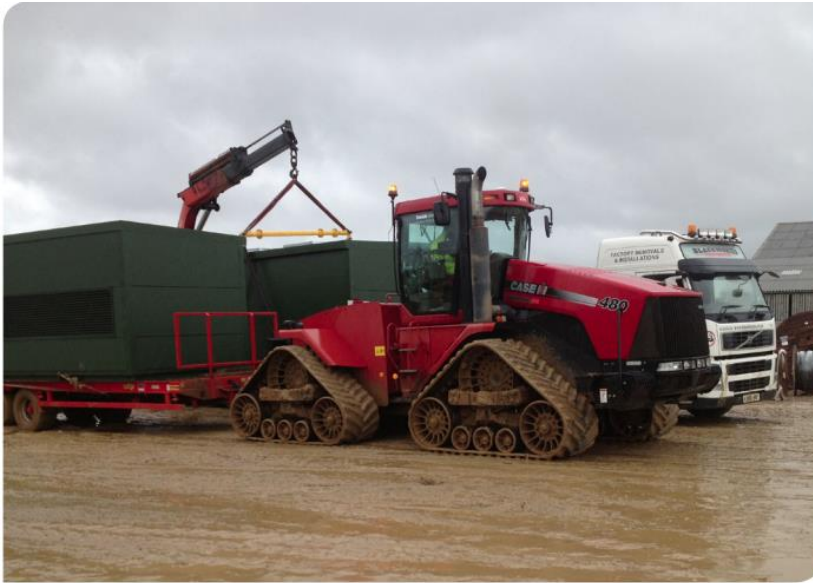
Case Steiger Quadtrac used to deliver inverters and other heavy equipment to site under soft ground conditions (photo courtesy of British Solar Renewables)
