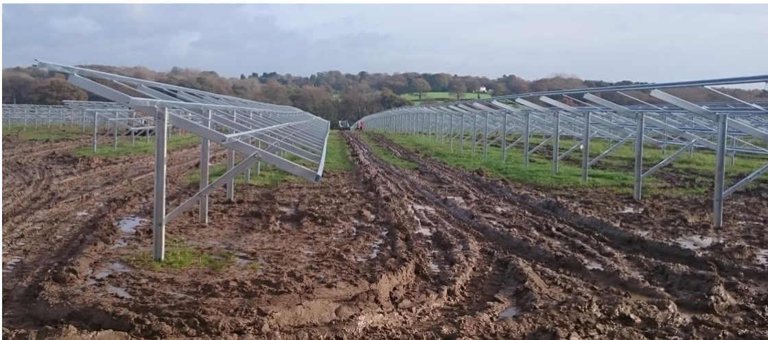
Inserts 8 and 9: Inter-row Ground Restoration
