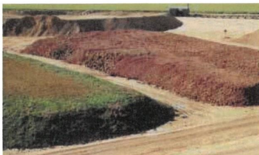
Clearly defined stockpiling of different soil materials
