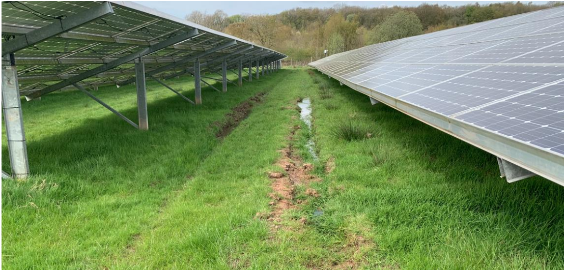
Insert 46: Deeper Rutting
